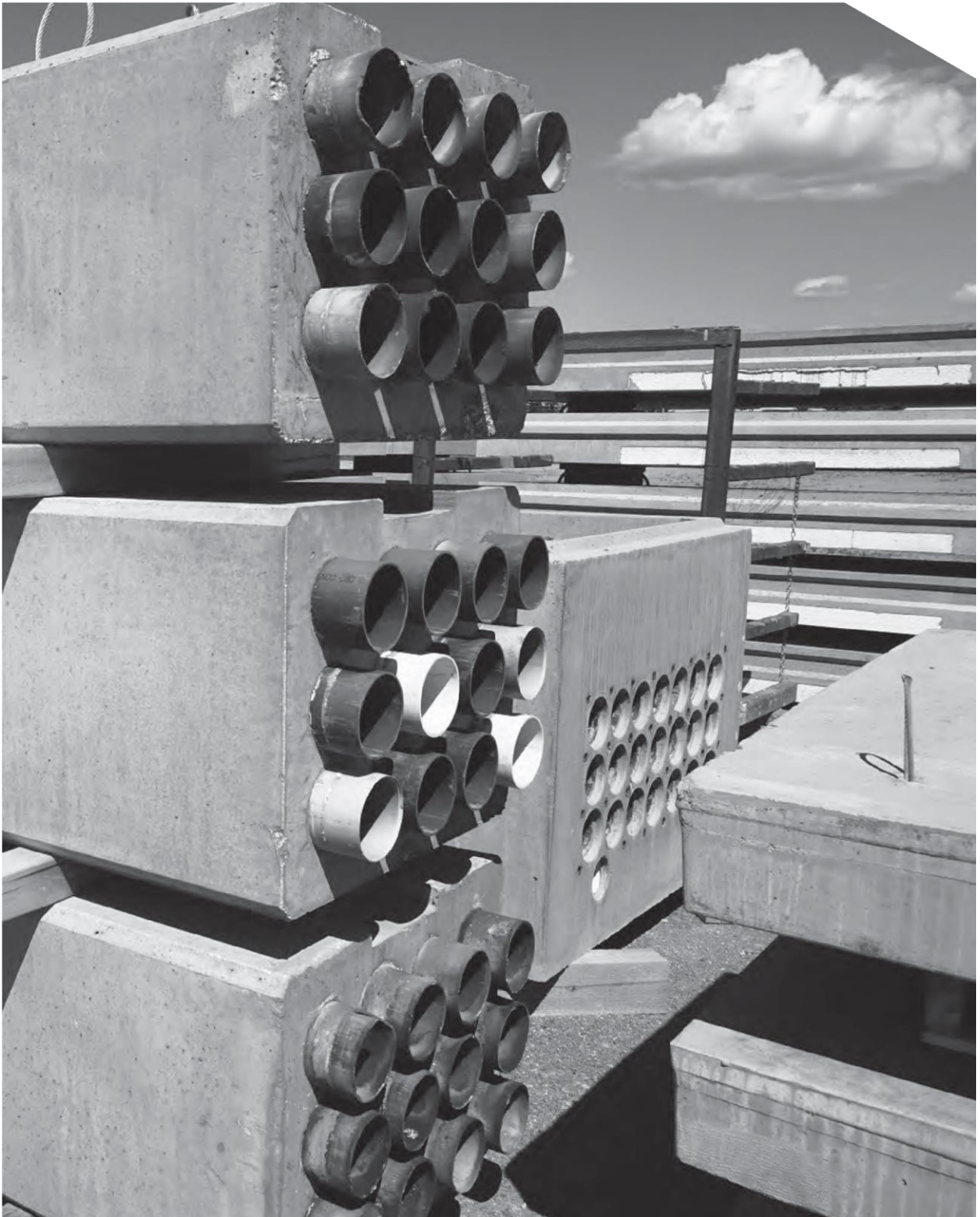
PRECAST 3x4 DUCT BANK
