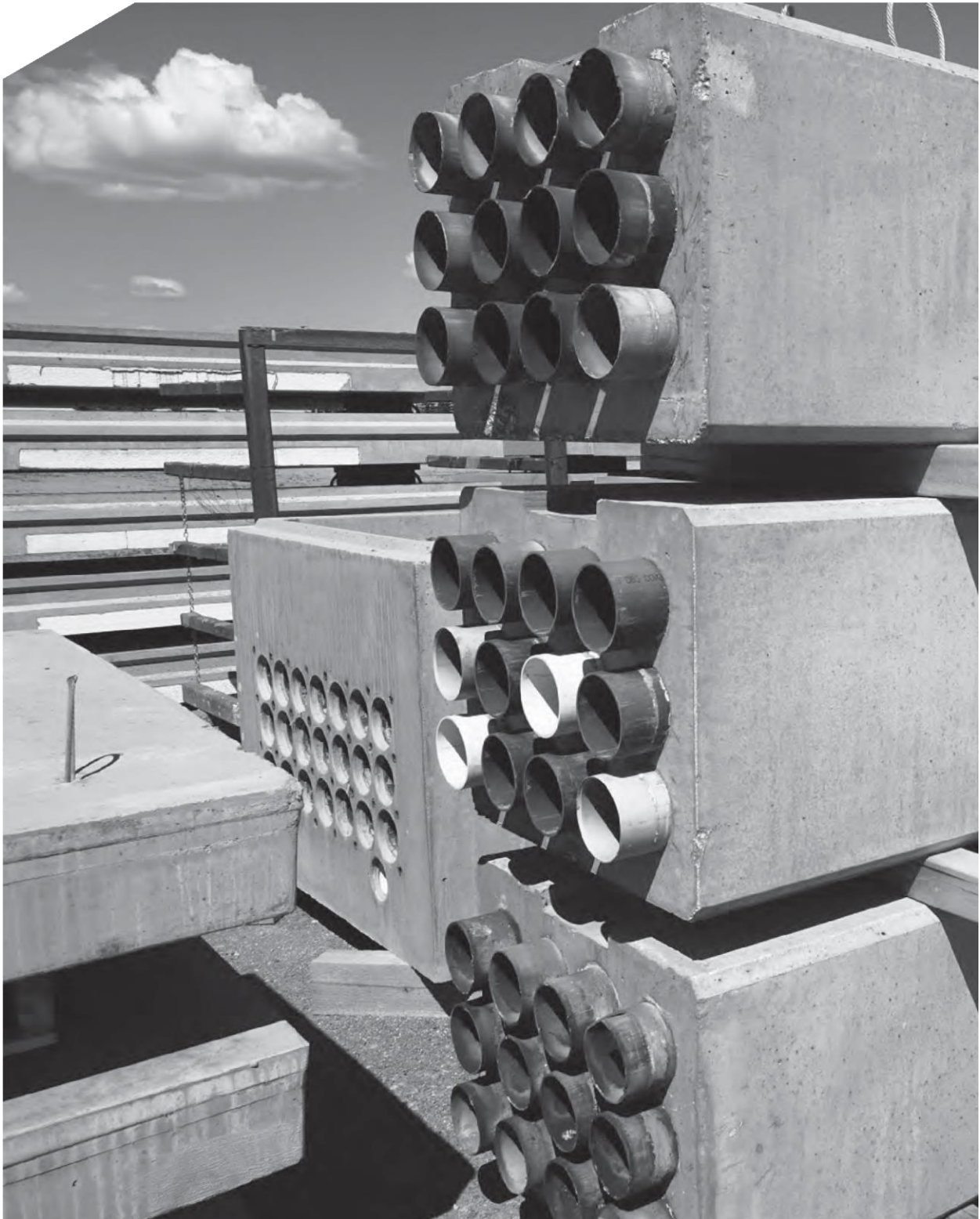
PRECAST 3x4 DUCT BANK
